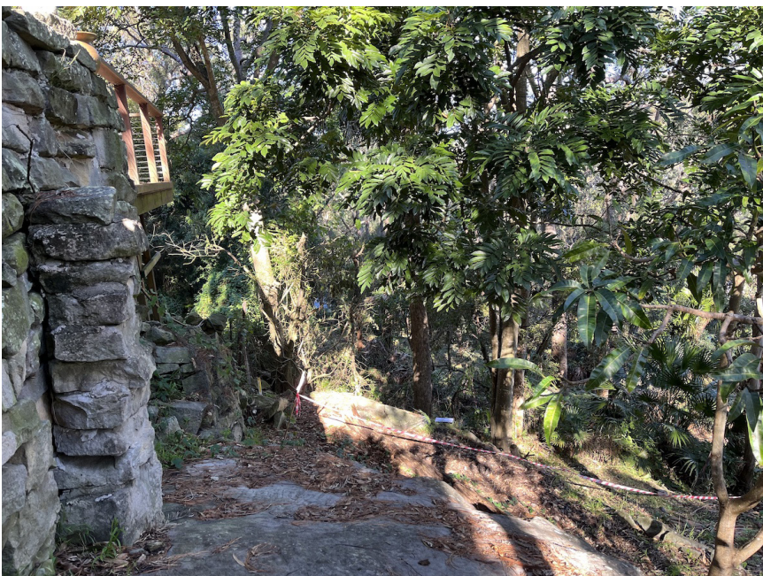
Figure 7 (left): Photograph viewing south along the eastern property boundary with the stone retaining wall visible to the left which is located on No. 60 Powderworks Road. (Photo: J Willis)
