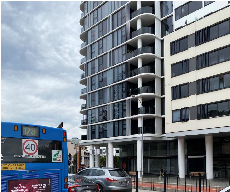
Photograph 3: Double height retail space created as part of the Meriton development, to provide a sense of space at the ground floor of the building, while allowing for additional natural light. A similar outcome is proposed for the development.
