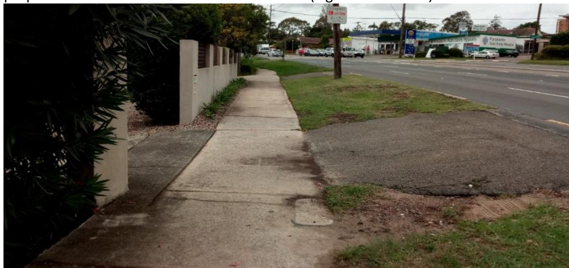
Figure 12. Driveway access and approximately 100mm high layback in front of No. 600 Warringah Road can be seen. Once gutter flow reaches 100mm it spills over the kerb and gutter crossing the layback into the property.
