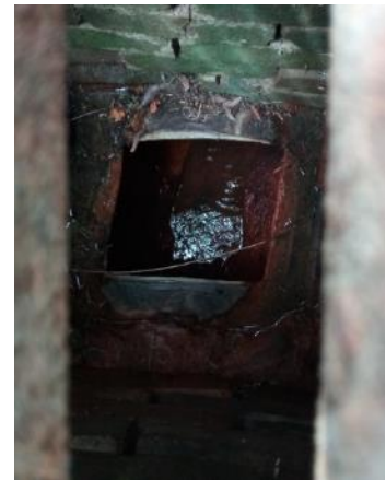
Figure 14 & 15. Existing surcharge pit next to the existing footpath can be seen in front of the site. There is an opening on top of the existing 600mm diameter pipe in the surcharge pit.
