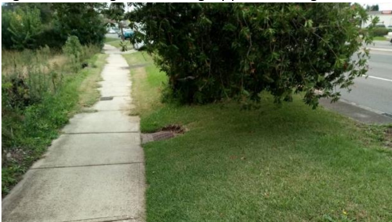
Figure 14 & 15. Existing surcharge pit next to the existing footpath can be seen in front of the site. There is an opening on top of the existing 600mm diameter pipe in the surcharge pit.
