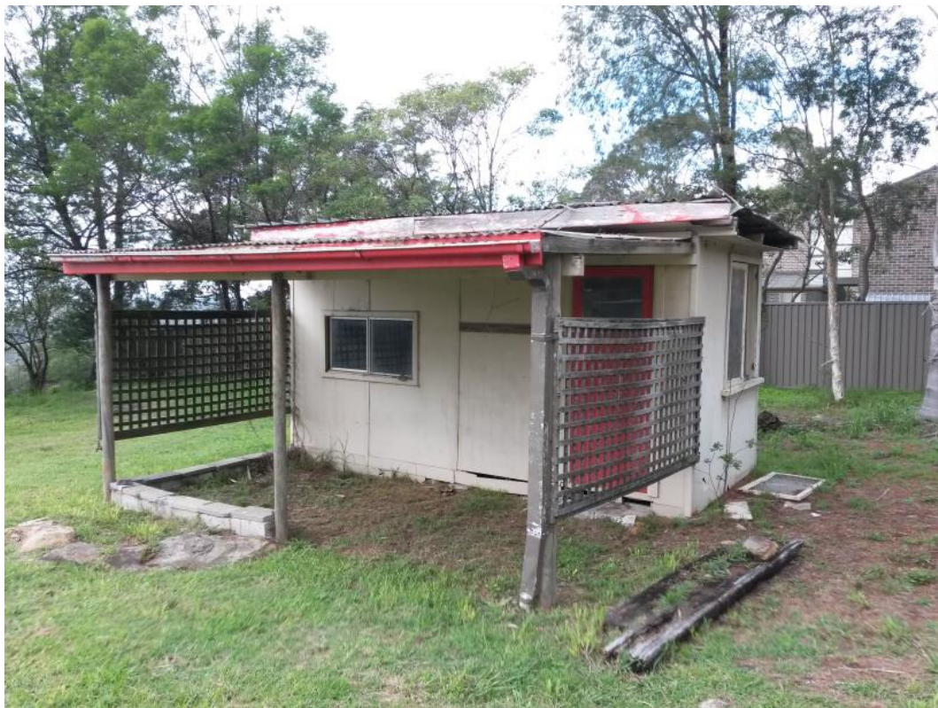
Figure 3: Building of Concern - Existing Shed ( confirmed to contain both asbestos containing materials and lead based paint – Appendix D ).
