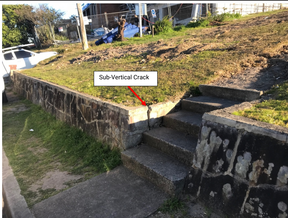
Photo 4 Sub-vertical crack discovered on the side of retaining wall.
