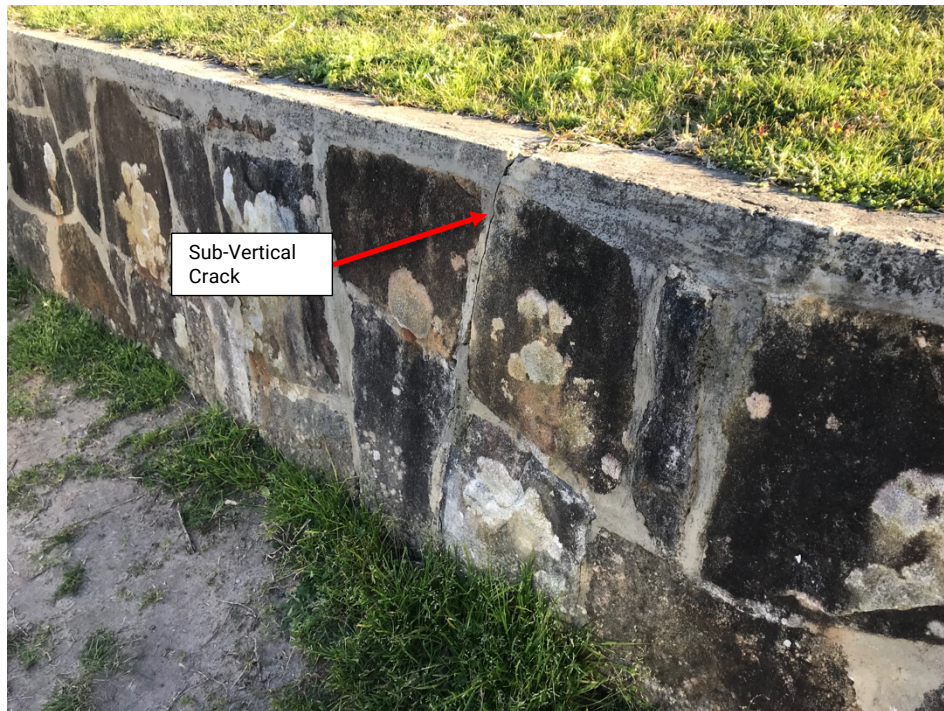
Photo 3 Sub-vertical crack discovered on retaining wall.
