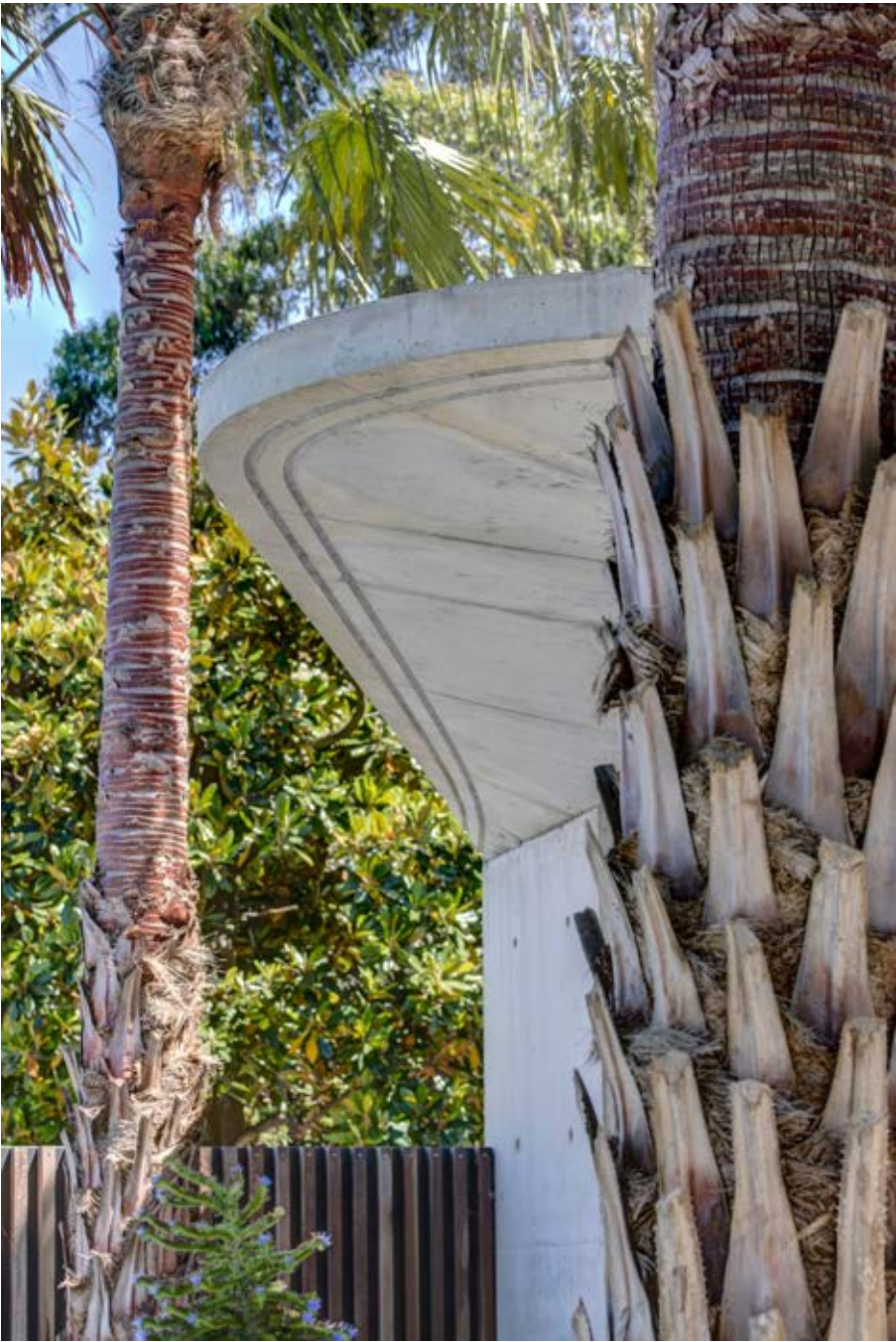
CONC _ NEW OFF-FORM CONCRETE
