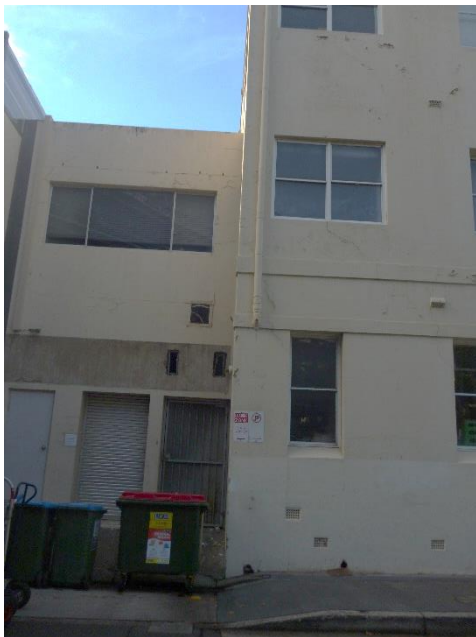
Figure 14: Rear (Market Place) elevation of 23 The Corso with the apartment building at 19-21 The Corso on the right.
