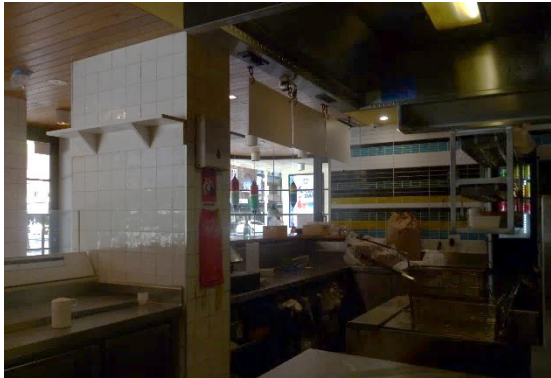
Figure 16: View of the kitchen area at the southern side of The Ivanhoe Hotel ground floor
