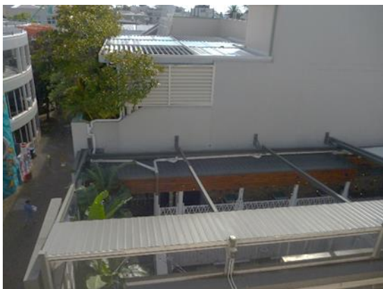
Figure 26: Rooftop view of 25 The Corso showing Market Place section
