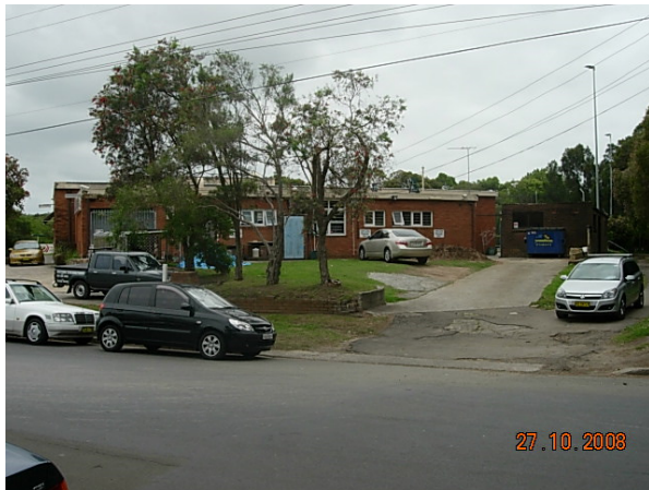
Photograph 1: Manly Vale Calabria Club as viewed from Campbell Parade.
