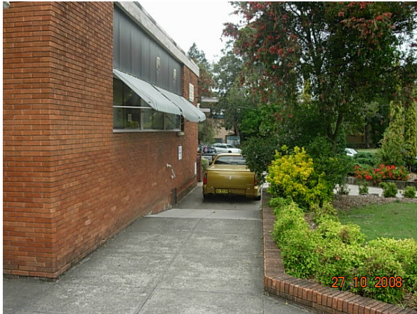
Photograph 3: Western elevation of building subject to the proposed extension.
