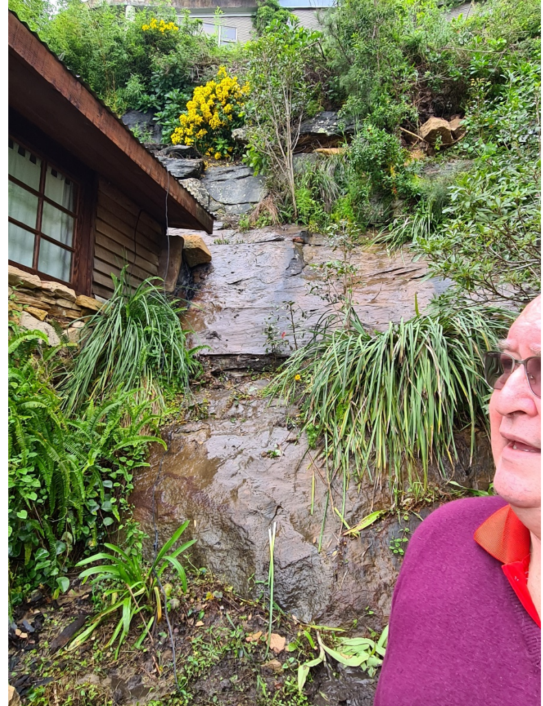
PHOTO 5 Block at rest against the secondary structure, 17 Florida Road.
