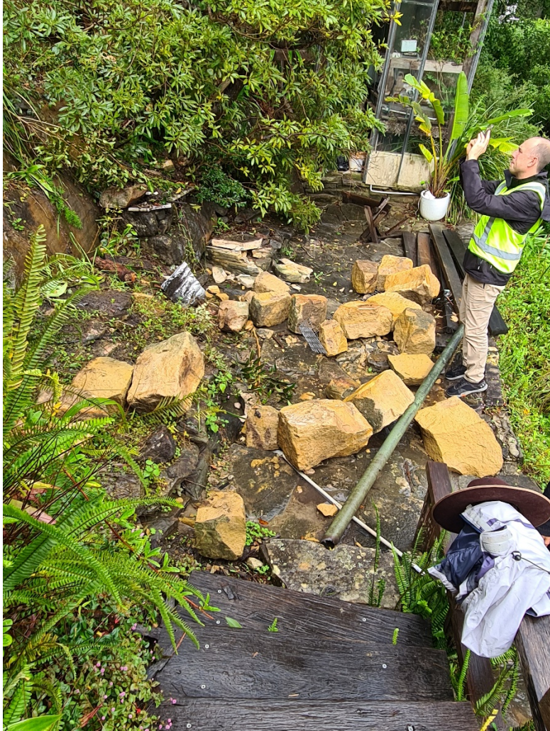
PHOTO 4 Sandstone block debris on flat sandstone bench at the rear of 17 Florida Road (Russell Peake in photo).
