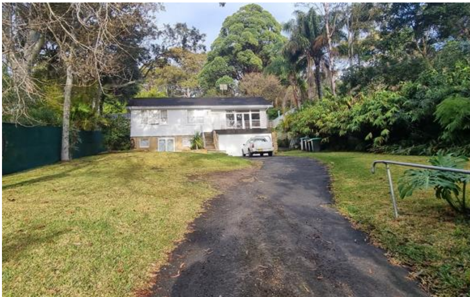
Photograph-3: View of front area of 27 Kevin Avenue. View looking south-west from the roadway.
