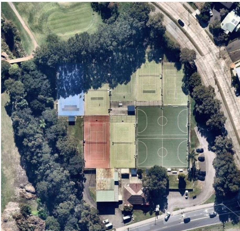
Figure 4: Site aerial (Source: www.nearmap.com )
