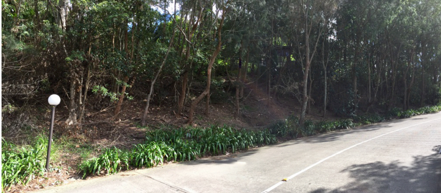
Cut batter on western side of internal access road
