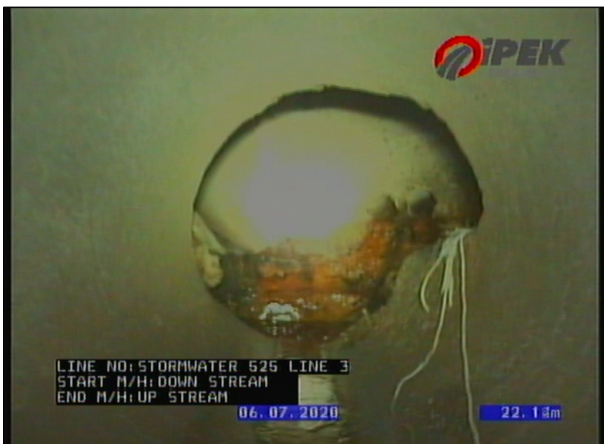
Photo: 6_11A 23.21m, Finish node, maintenance hole, Nodename: SPP01247
