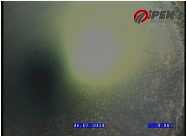
Photo: 2_1A 0m, Start node, maintenance hole, Nodename: SPP01246
