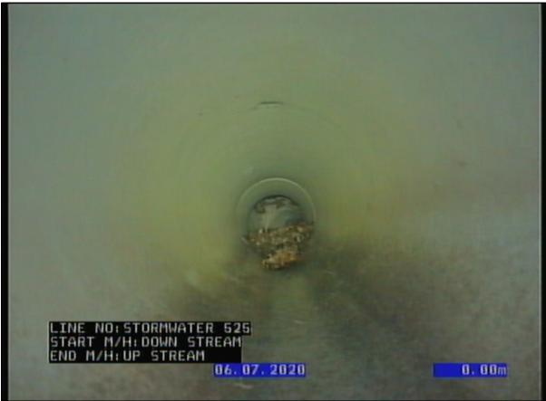
Photo: 4_1A 0m, Start node, maintenance hole, Nodename: SPP01246
