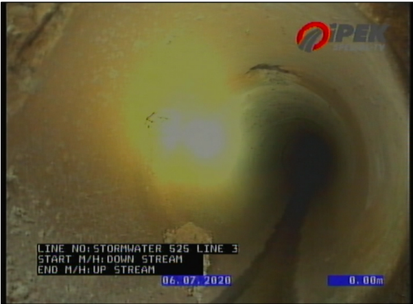
Photo: 6_1A 0m, Start node, maintenance hole, Nodename: SPP04649
