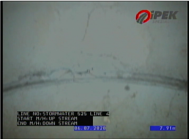
Photo: 4_3B 7.91m, Breaking, all pieces are present but some of them are visibly displaced from position, length of break 100 , from 10 to 1 o'clock
