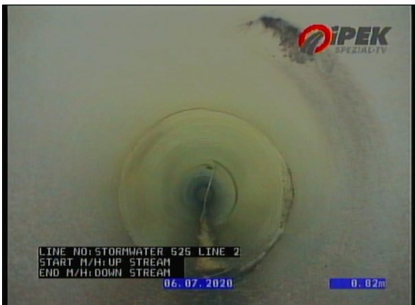
Photo: 2_3A 1.66m, Breaking, all pieces are present but some of them are visibly displaced from position, length of break 100 , from 12 to 12 o'clock
