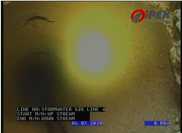
Photo: 4_1A 0m, Start node, maintenance hole, Nodename: SPP04649
