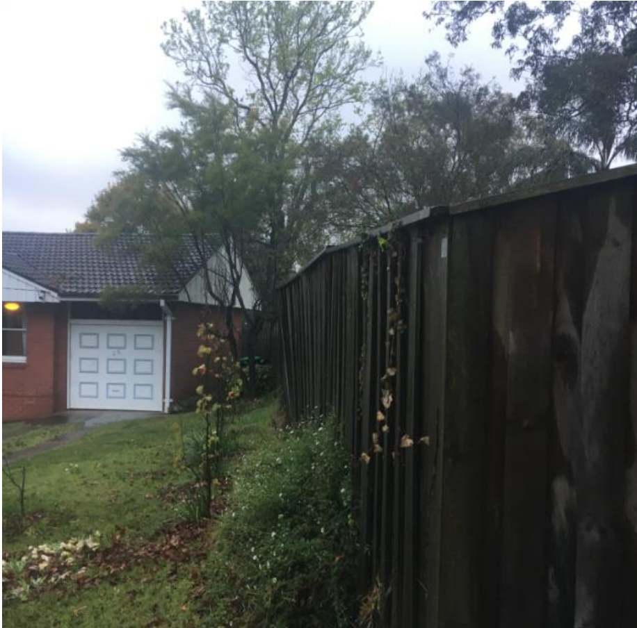
Photo showing boundary fence located inside our property line with substantial lean
