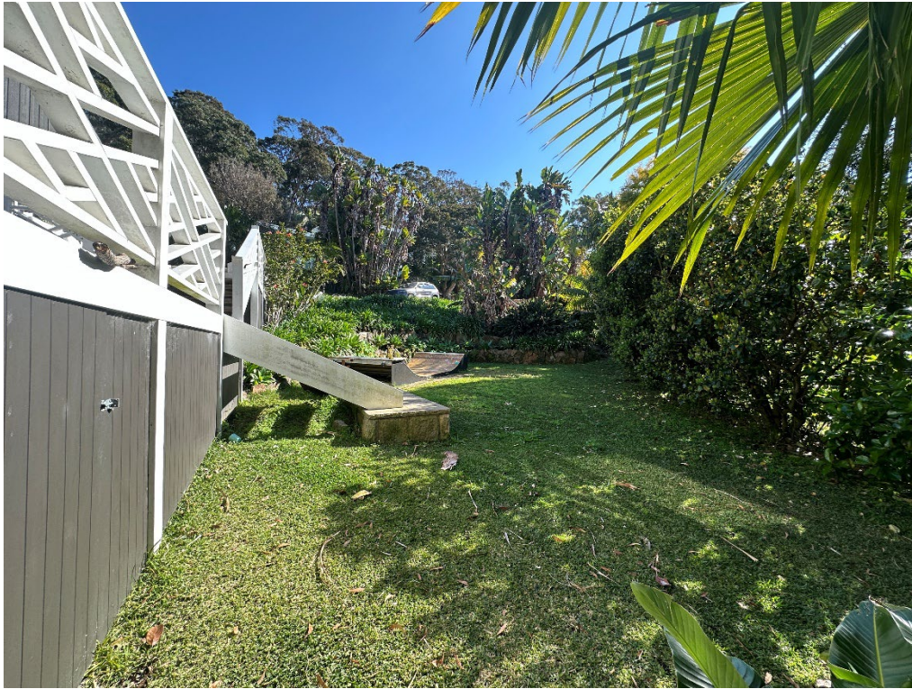
Figure 5. View of proposed position of pool, set into the garden area (beyond stairs)
