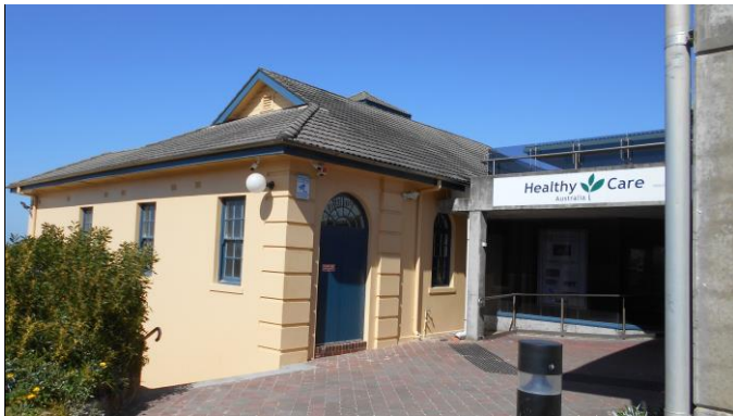
Entry doors and infill section between original and 1980s section of the building
