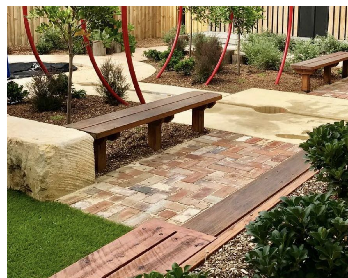
Recycled brick Paving
