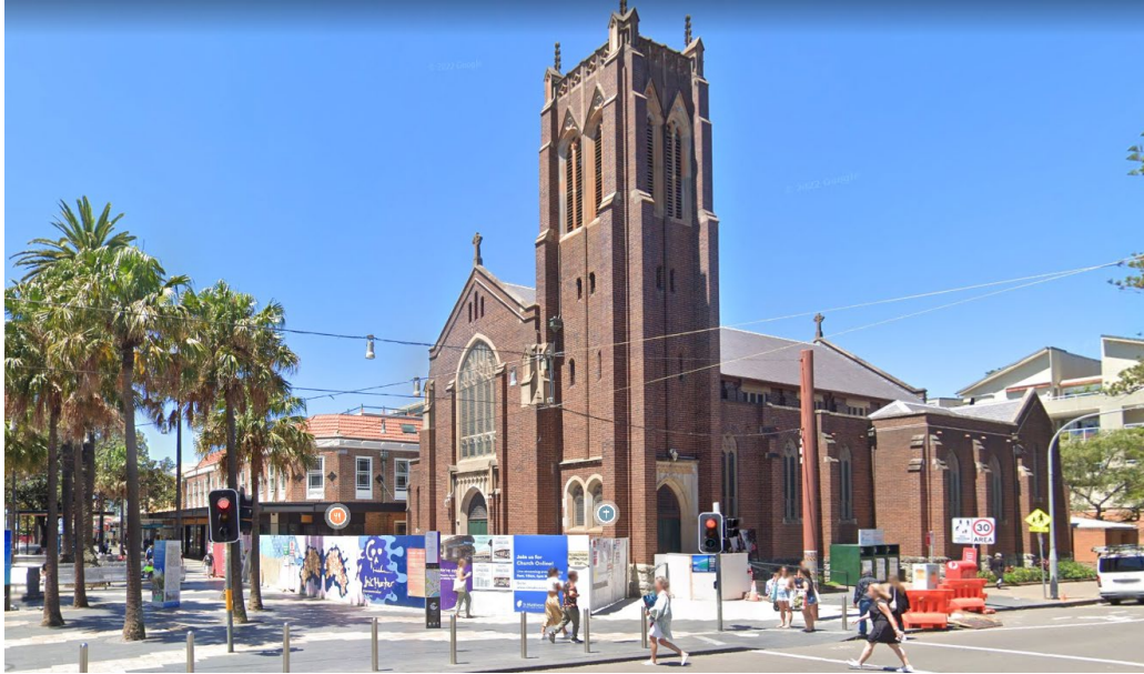
Figure 9: St Matthews Manly, located on the southern side of The Corso, opposite the site, at 1 Darley Road
