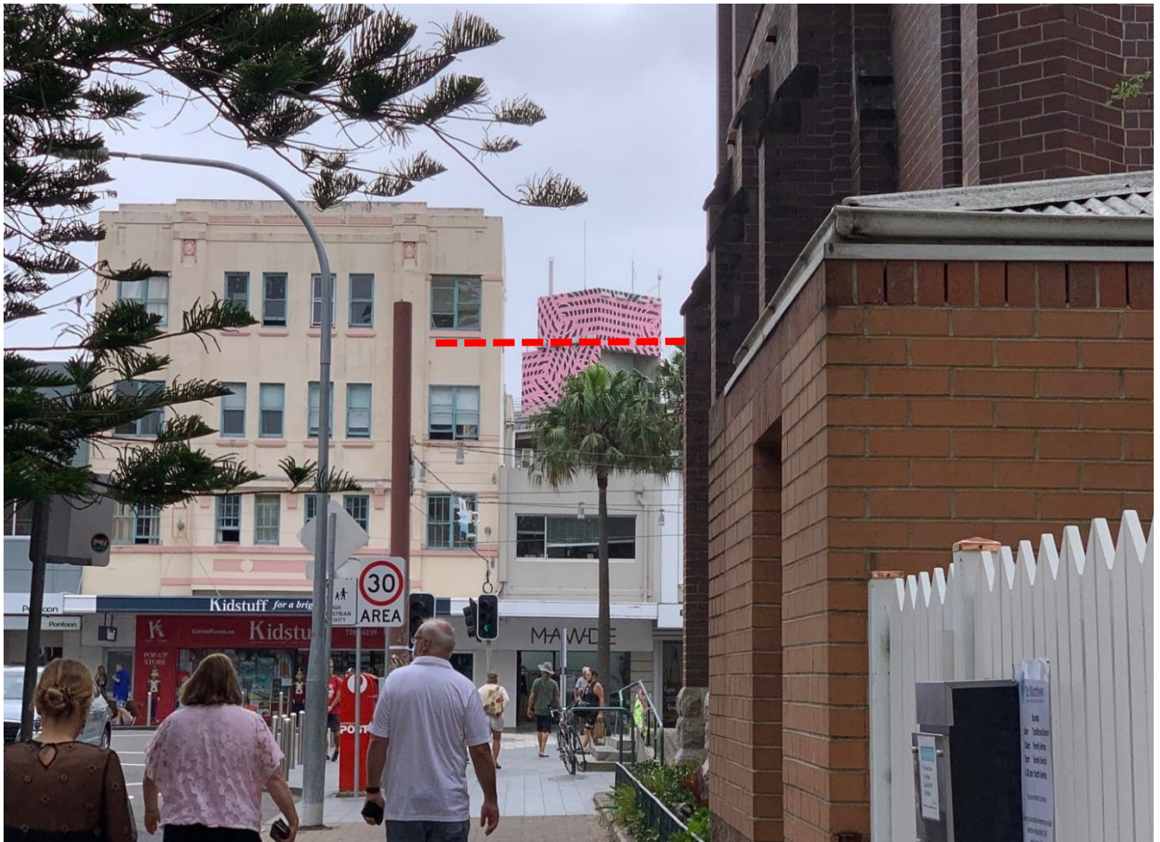
Photograph 1: View of Market Lane car park from Darley Lane, looking north and approximate sill height transposed across No. 23
