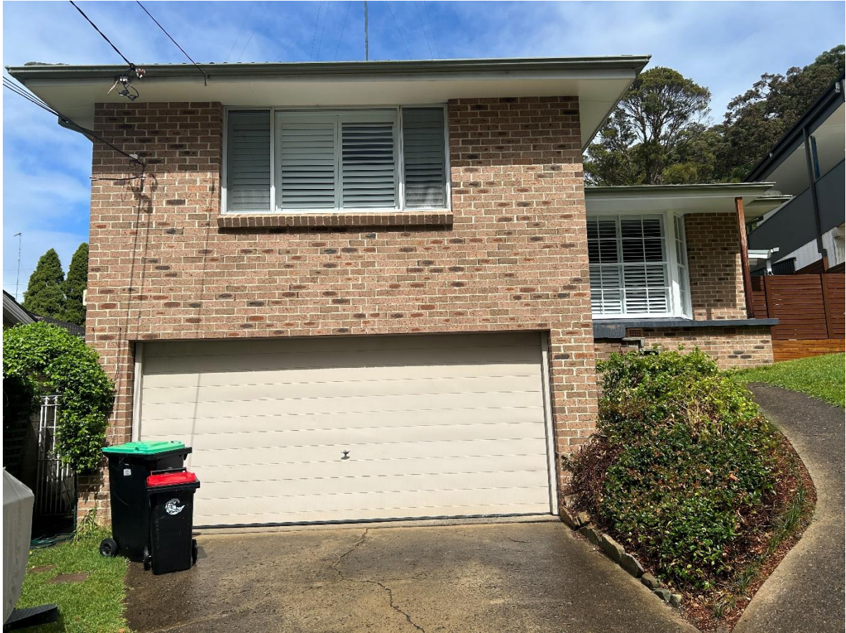
Figure 4: Front façade of the dwelling with proposed first floor above.
