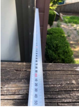
Picture taken of measurement of proposed fire egress path less than 1m.
