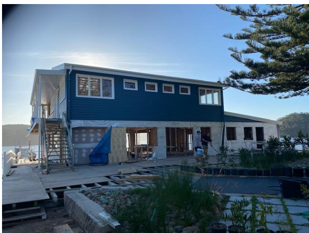
Figure 2: The new replacement Boathouse café building under construction with powder coated aluminum window and door leaves framed in with timber architraves and reveals.
