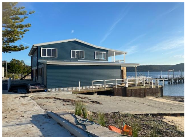
Figure 2: The new replacement Boathouse café building under construction with powder coated aluminum window and door leaves framed in with timber architraves and reveals.
