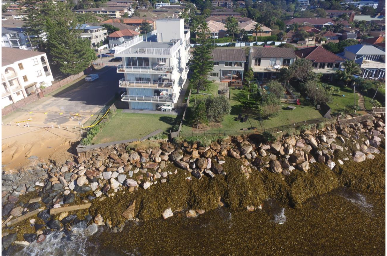
Figure 10: Erosion and damage at 1172 and subject properties 1174, 1176 and 1178 on 10 June 2016, with damage to fences and backyard erosion at all properties
