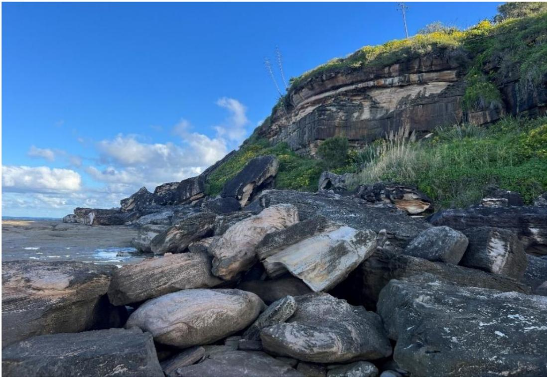
**Figure 4-3 Boulder armour at the cliff toe**
