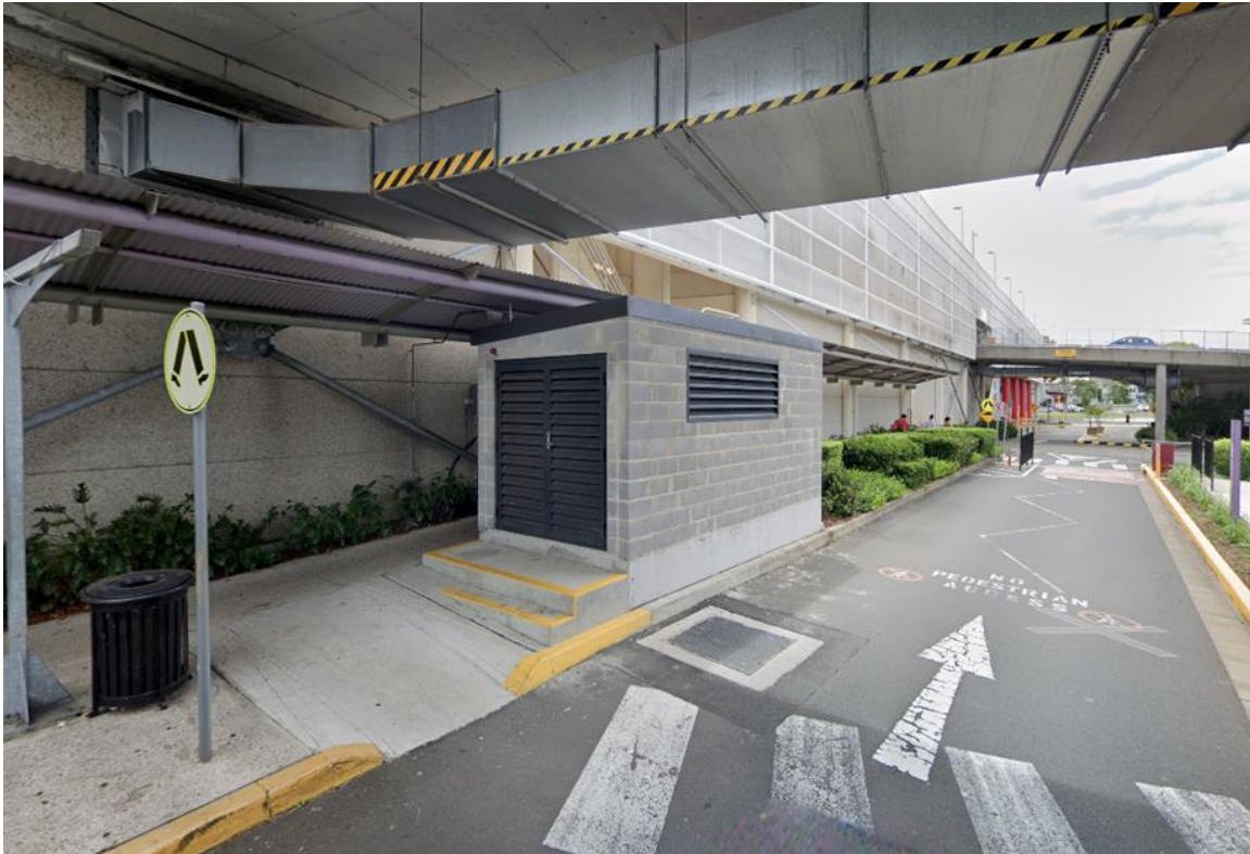
Figure 3 – Existing Brick Structure Housing Sewer Station
