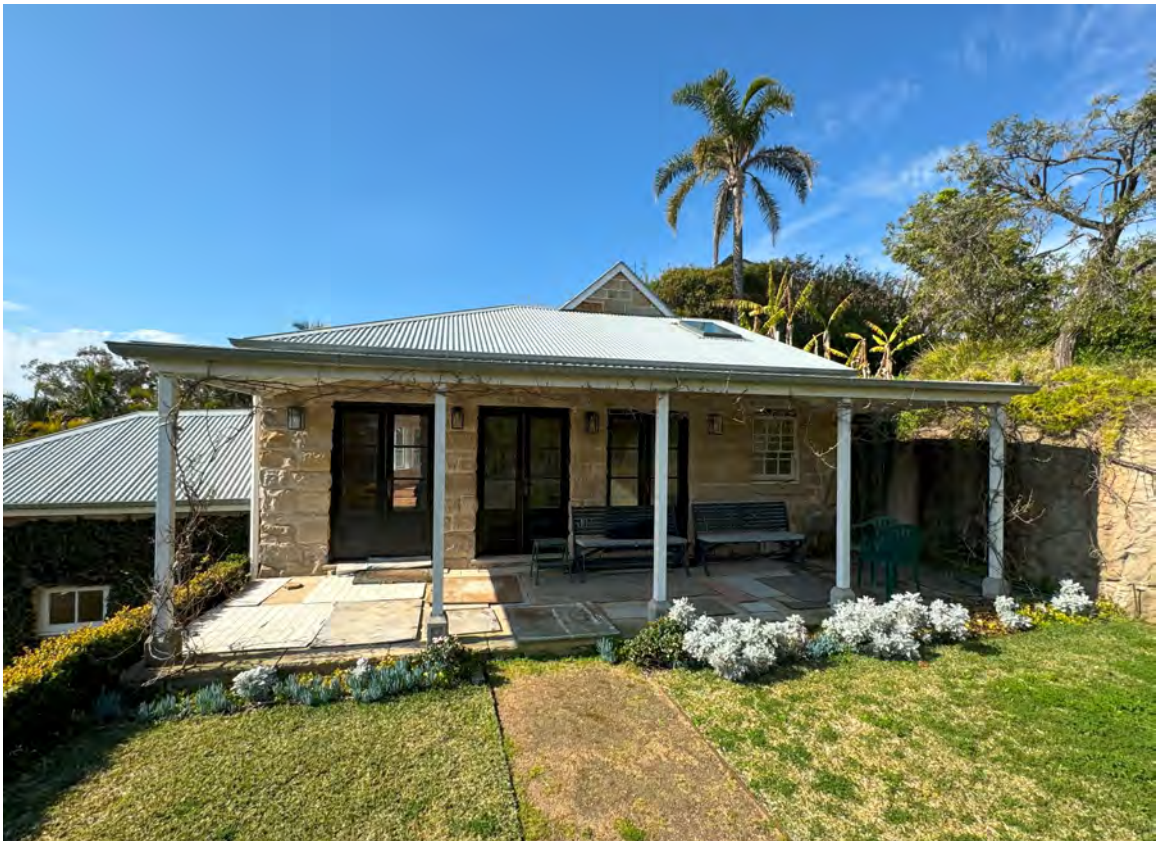
West elevation—verandah is an addition, as are three French door openings.
