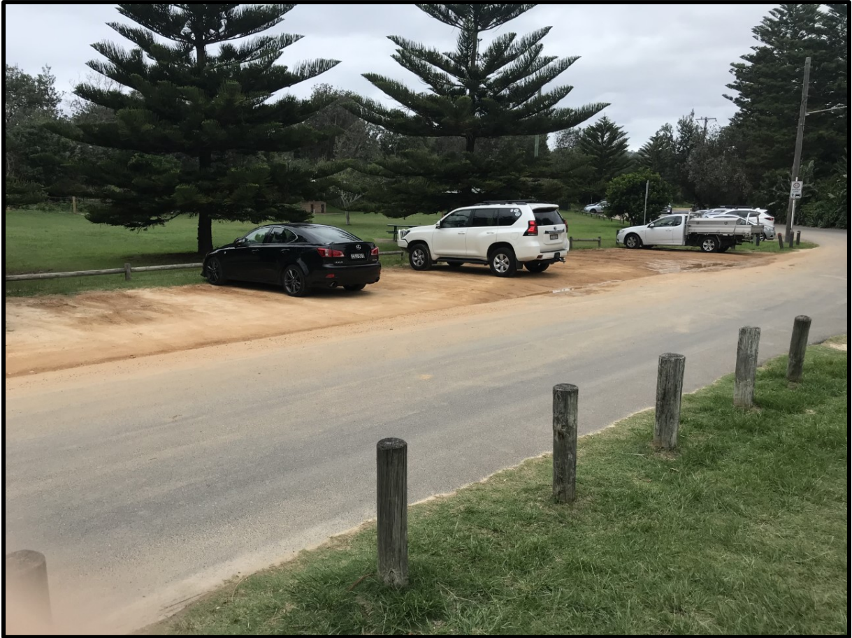
SUBJECT CARPARK, NOTE WATER RETENTION AND SEDIMENT ON ROADWAY
