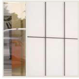
1 Translucent glass structurally glazed onto aluminium framing
