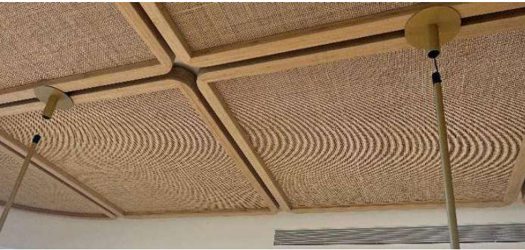
NEW RATTAN INSERTS TO EXISTING CEILING COFFERS (OFFSET TO EXPOSE EXISTING CORNICES)
