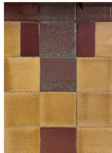
EXISTING TILES TO WALLS TO BE RETAINED AND MADE GOOD
