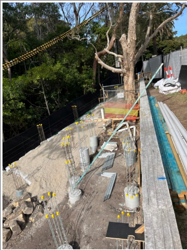
Figure 1 Shows the piers within the TPZ of Tree 2.
