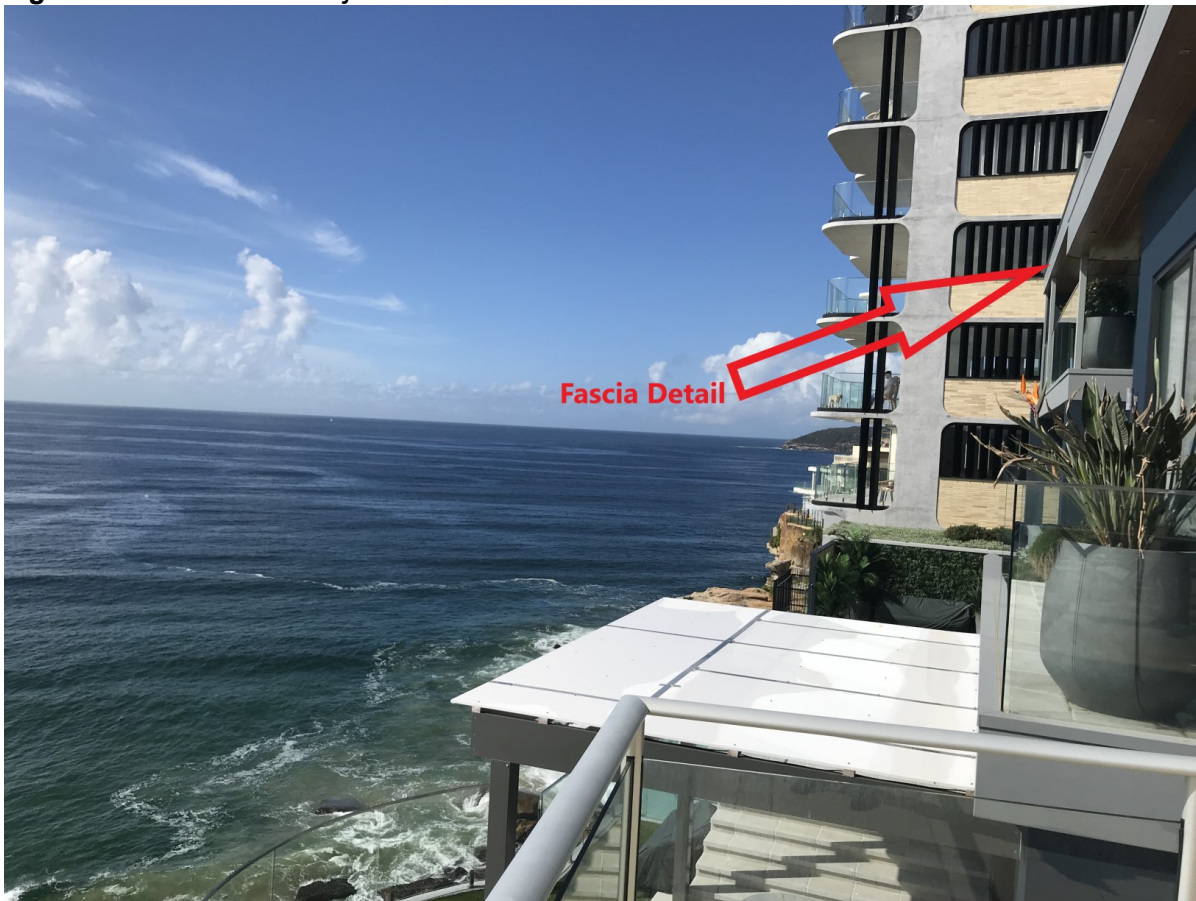
Figure 7: fascia detail subject to this modification when viewed from 9 Pavilion Street
