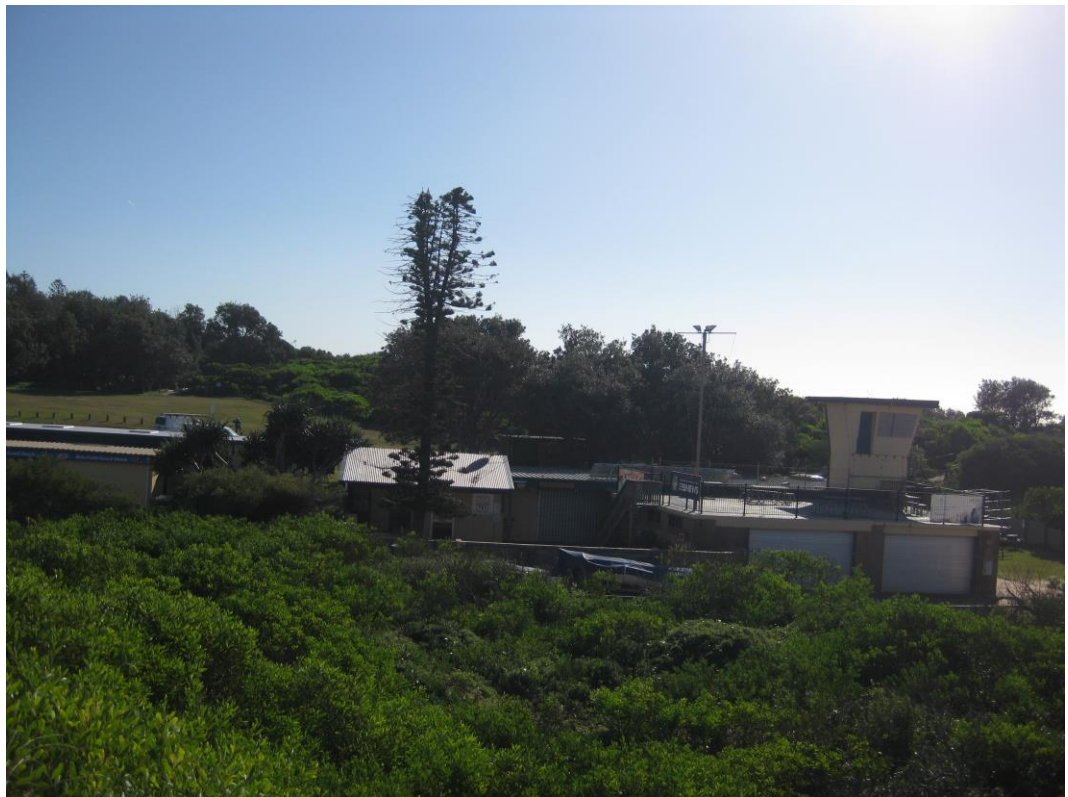
Figure 4 Existing Long Reef SLSC building and amenities block as viewed from the dunes to the south.
