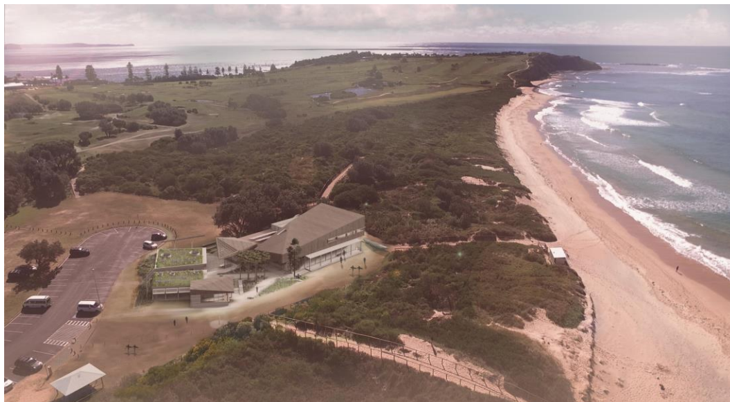
Figure 9 Aerial view of the three new buildings.
