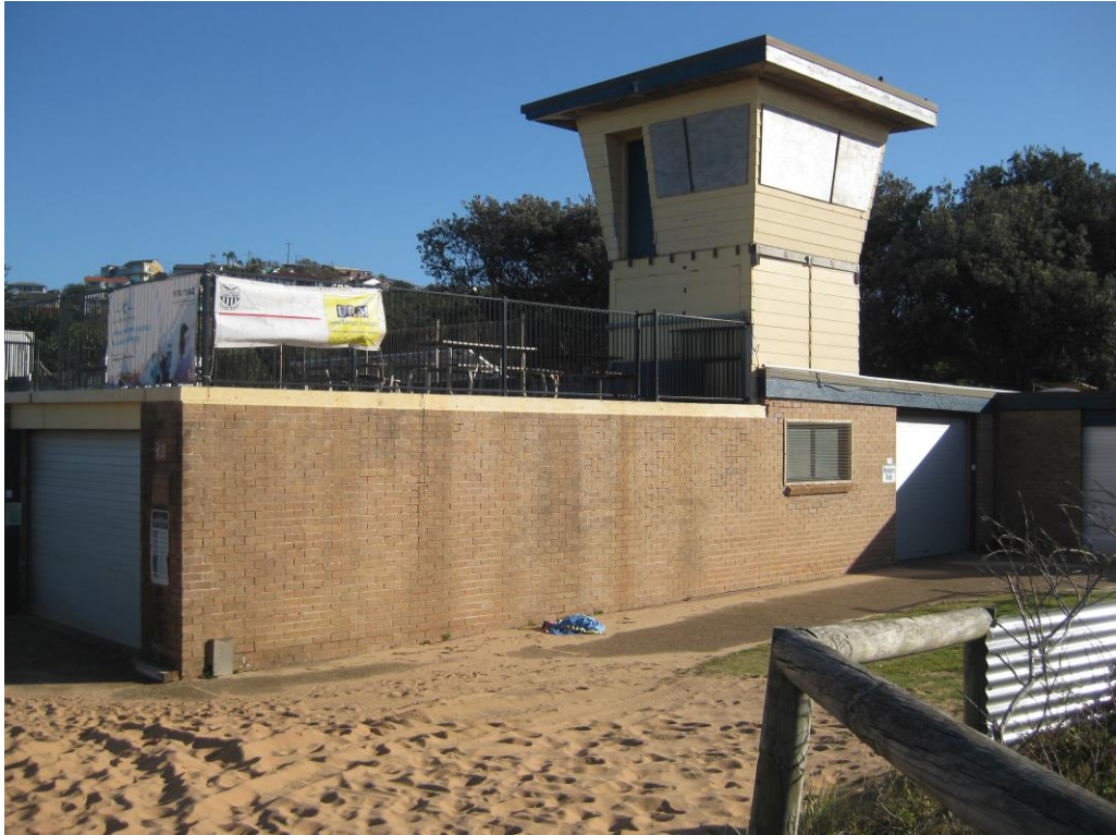
Figure 5 Existing LRSLS building with tower and rooftop terrace
