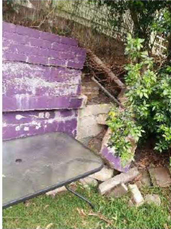
Figure 2 Partial view of the damaged boundary retaining wall
