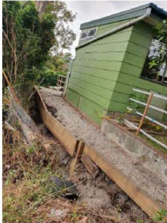
Figure 3 Partial view of damaged boundary retaining wall, including neighbouring property
