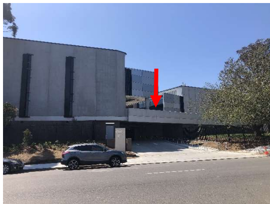
Figure 10: View of Northern Beaches Business Park from South Creek Road, opposite the entry to the basement carpark, with the location of the subject tenancy marked with an arrow
