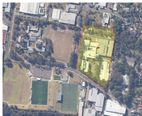
Figure 2: Aerial view showing 4-8 Inman Road, Cromer, outlined in red and coloured yellow. Note this image was taken prior to the approved redevelopment of the site and does not show the new building that is the subject of this report. (Source: Source: Sixmaps)
