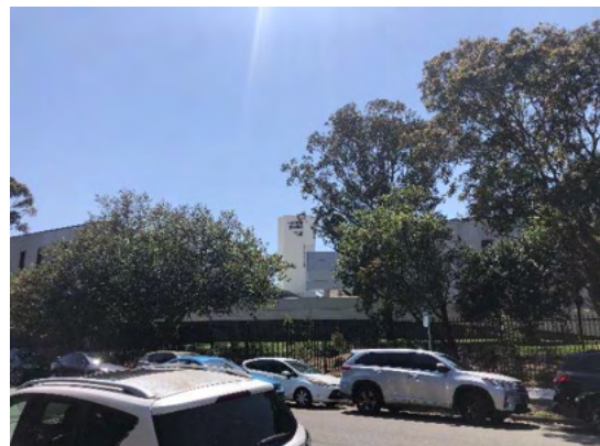
Figure 11: View of Northern Beaches Business Park from east of the carpark entry showing the retained hexagonal tower from the Roche Complex
