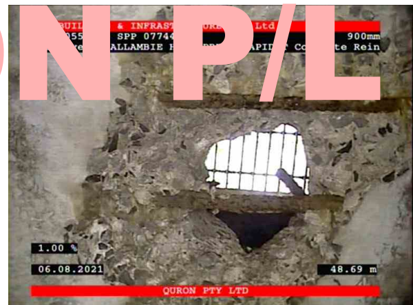
16, 00:17:11, 48.69 Reinforcement is exposed and corroded at 12 o'clock
