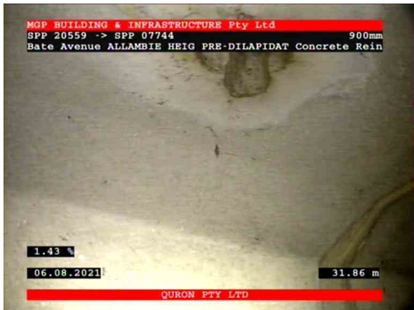
9, 00:10:42, 31.86 Connection, poor workmanship, connection appears to be open, height: 200mm at 12 o'clock
