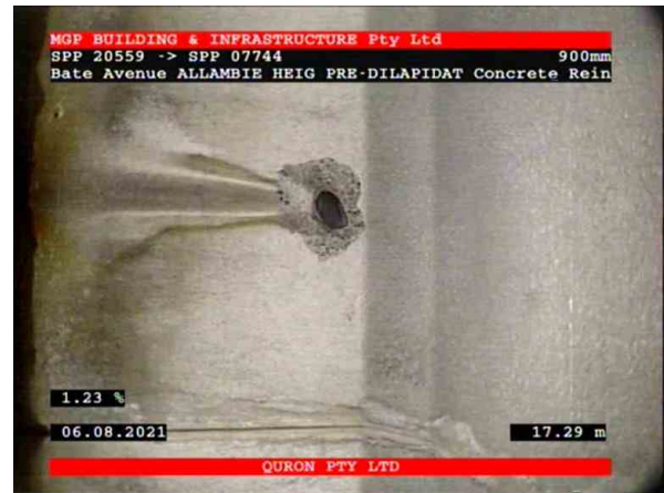
2, 00:04:45, 17.29 Connection, good workmanship, connection appears to be open, height: 100mm at 10 o'clock
