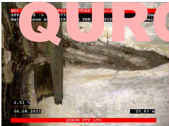
3, 00:07:04, 25.83 Tap roots--a small number of major roots (10mm or greater) without a significant mass of fine root, at joint, Obstruction: <5% at 8 o'clock
