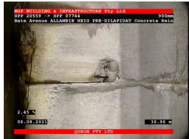
6, 00:09:30, 30.96 Connection, poor workmanship, connection appears to be open, height: 100mm at 10 o'clock
