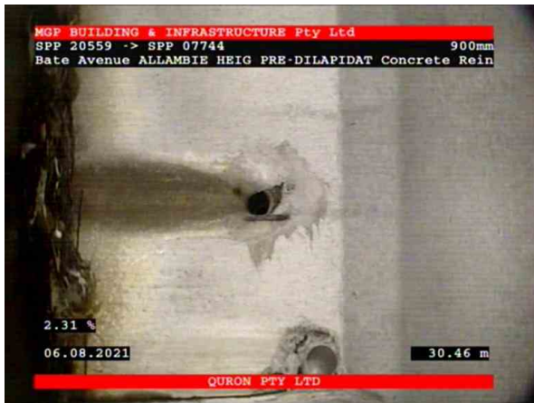
5, 00:09:16, 30.46 Connection, poor workmanship, connection appears to be open, height: 100mm at 9 o'clock
