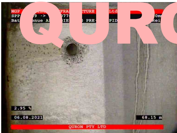
19, 00:24:37, 68.15 Connection, good workmanship, connection appears to be open, height: 100mm at 9 o'clock
