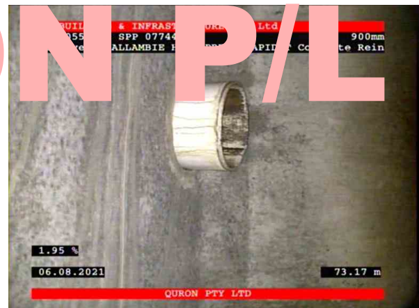
20, 00:30:12, 73.17 Intruding connection, magnitude of intrusion: <5% at 12 o'clock
