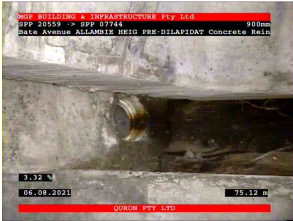
21, 00:30:51, 75.12 Connection, good workmanship, connection appears to be open, height: 100mm at 2 o'clock
