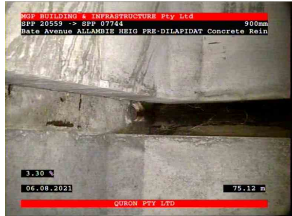
22, 00:30:51, 75.12 Connection, good workmanship, connection appears to be open, height: 100mm at 2 o'clock
