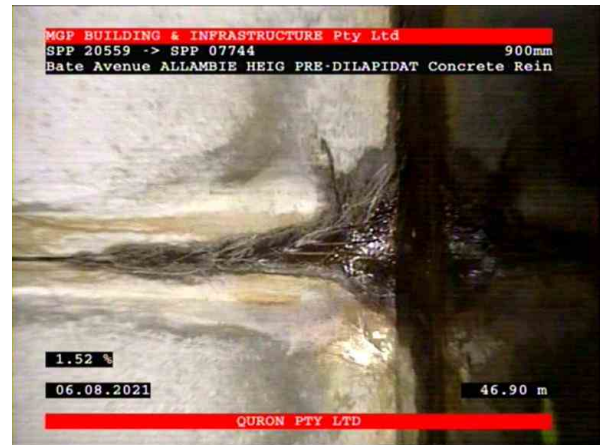
14, 00:16:38, 46.90 Fine roots--a relatively small number of flexible minor roots, at joint, Obstruction: <5% from 3 o'clock to 4 o'clock
