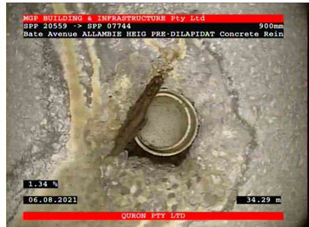
10, 00:13:35, 34.30 Connection, poor workmanship, connection appears to be open, height: 100mm at 12 o'clock
