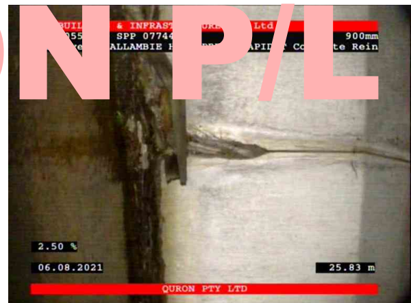
4, 00:07:04, 25.83 Tap roots--a small number of major roots (10mm or greater) without a significant mass of fine root, at joint, Obstruction: <5% at 8 o'clock
