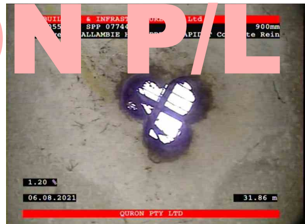
8, 00:10:42, 31.86 Connection, poor workmanship, connection appears to be open, height: 200mm at 12 o'clock
