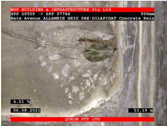
17, 00:19:41, 53.19 Connection, poor workmanship, connection appears to be open, height: 150mm at 12 o'clock
