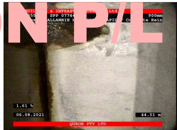
12, 00:16:03, 44.51 Connection, good workmanship, connection appears to be open, height: 100mm at 9 o'clock
