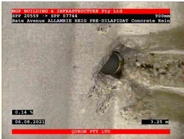
1, 00:00:48, 3.25 Connection, poor workmanship, connection appears to be open, height: 100mm at 2 o'clock
