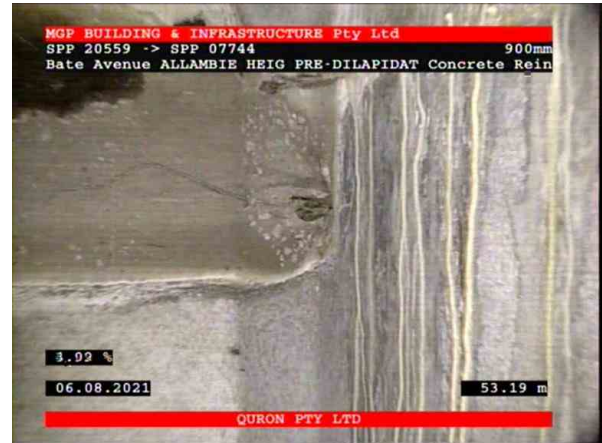
18, 00:19:41, 53.19 Connection, poor workmanship, connection appears to be open, height: 150mm at 12 o'clock
