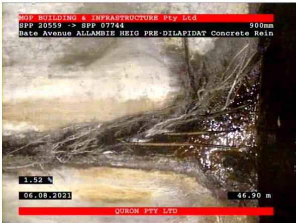
13, 00:16:38, 46.90 Fine roots--a relatively small number of flexible minor roots, at joint, Obstruction: <5% from 3 o'clock to 4 o'clock
