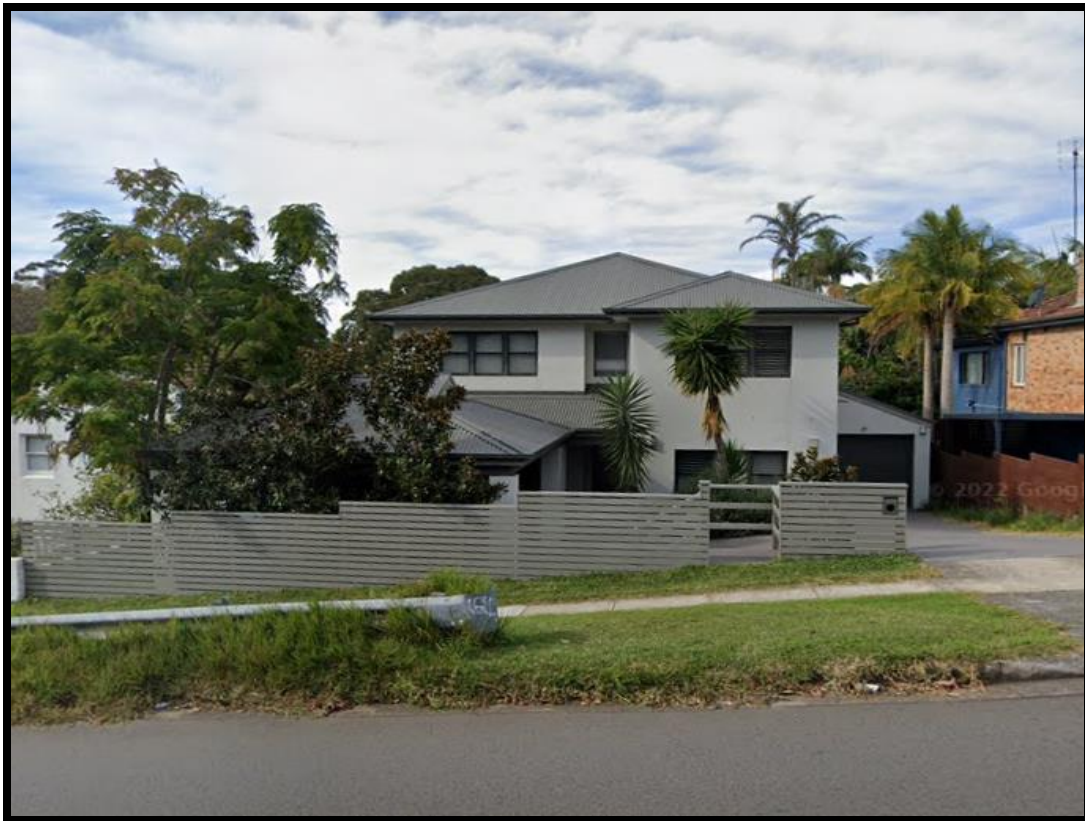
View of the adjoining northern property – No 8 Redman Street
