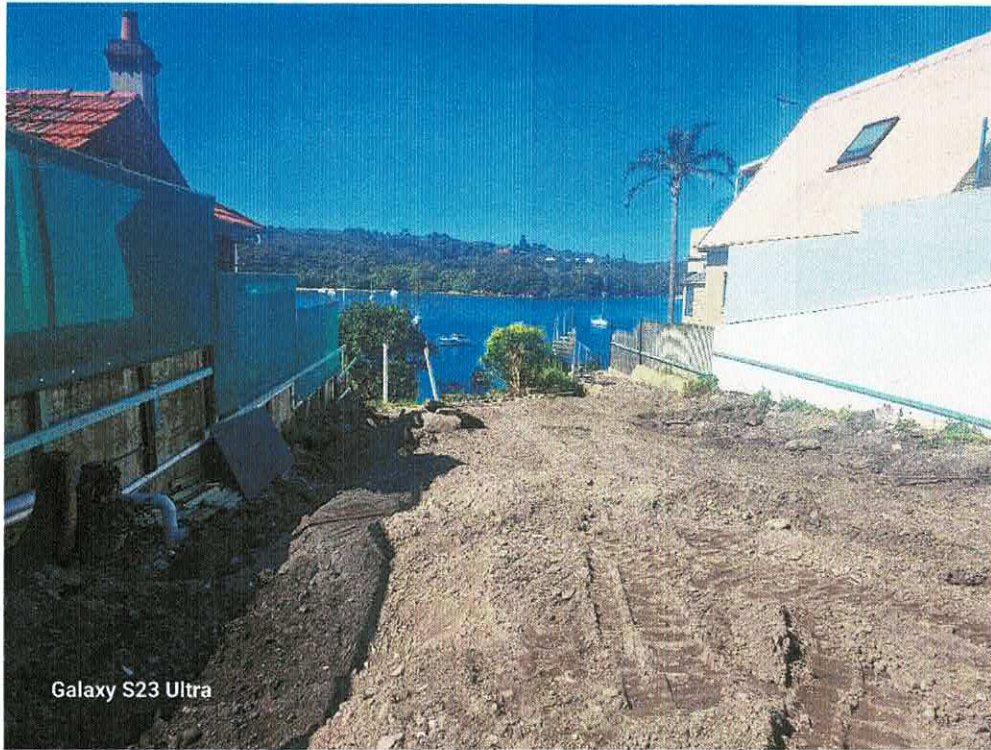
Photograph 9: Existing dwelling demolished cleared site
