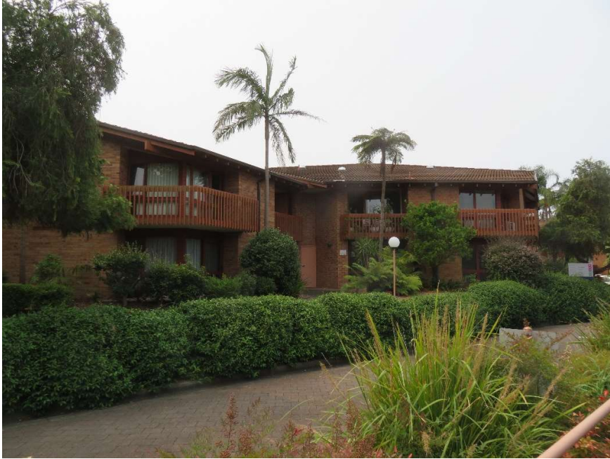
Photo 4: South Western facade
