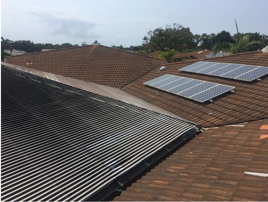
Photo 2: Adjacent rooves to the proposed works
