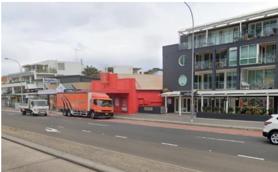
Figure 6 - Photograph of the 4 storey shop top housing development located along Pittwater Road to the north and south of the subject site
