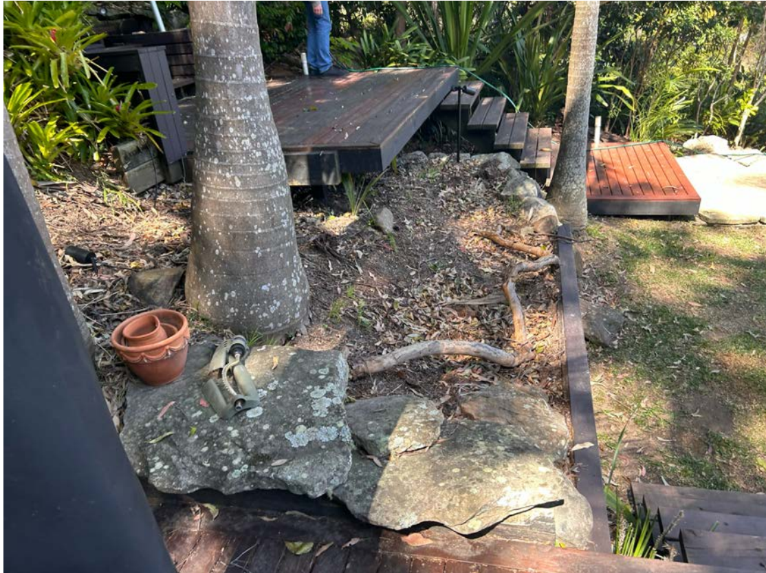
Figure 5: Rear Retaining Wall (Source: JS Urban Design)
