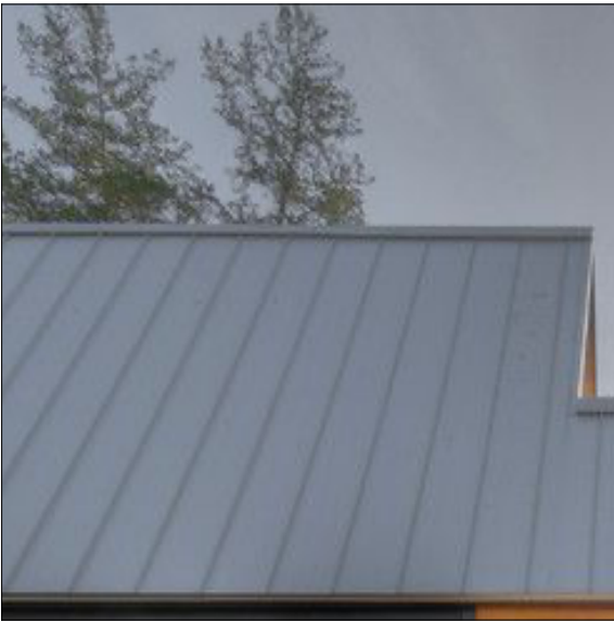
RF - 01 - Metal deck roof
