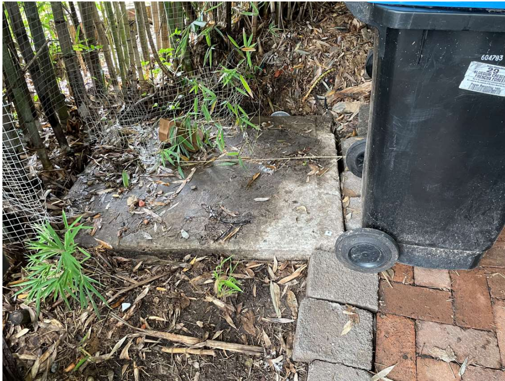
Figure 4: Existing stormwater pit SSP01245 (Solid lid)
