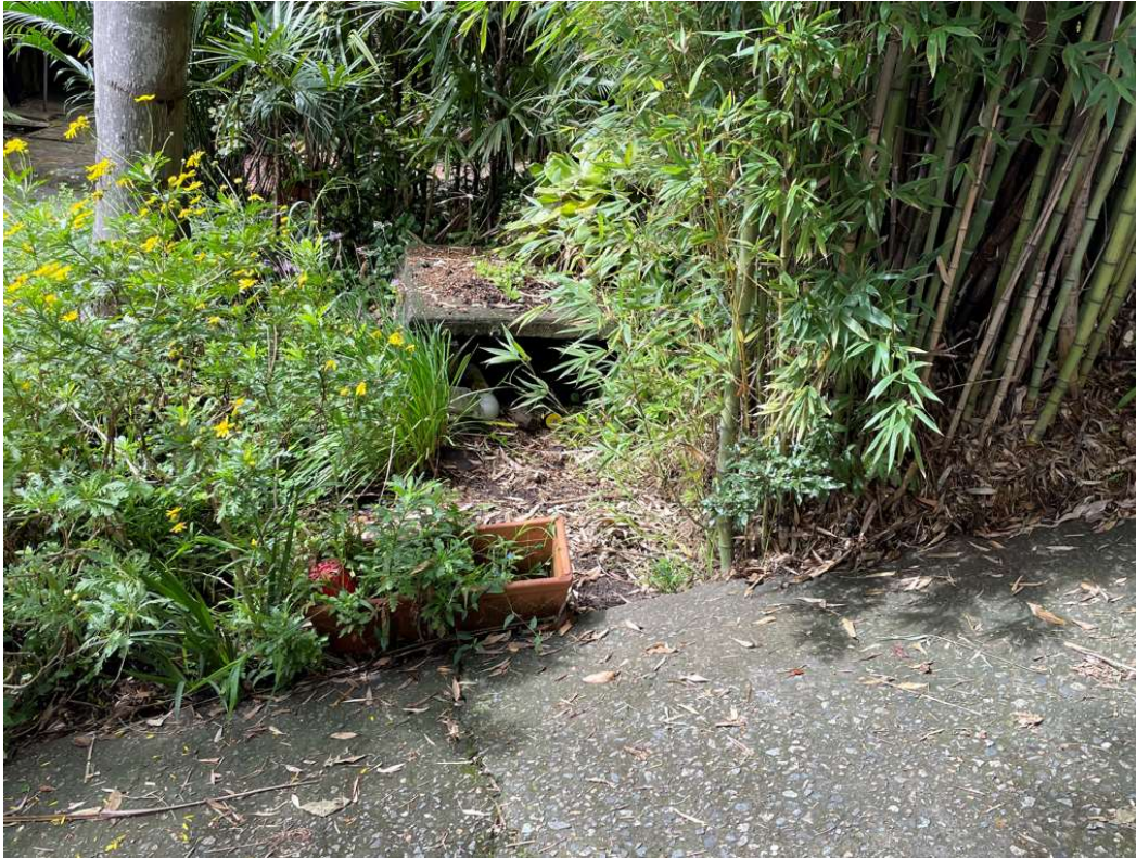
Figure 6: Existing stormwater pit SSP01246
