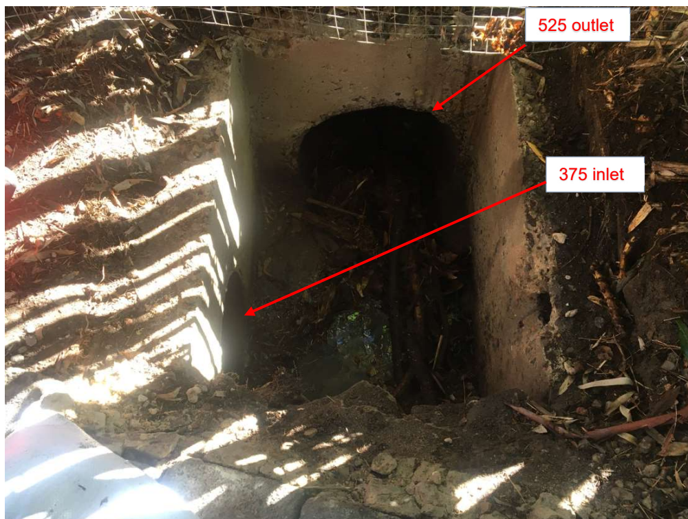
Figure 5: Existing stormwater pit SSP01245
