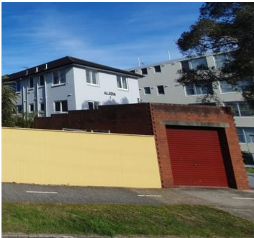
Photograph 6 – View of the front brick garage, looking south from the roadway.
