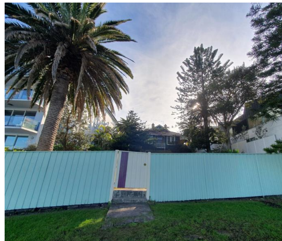
Photograph 3 – Rear view of the property with a rear colorbond fence, looking north from Fairlight Beach area.
