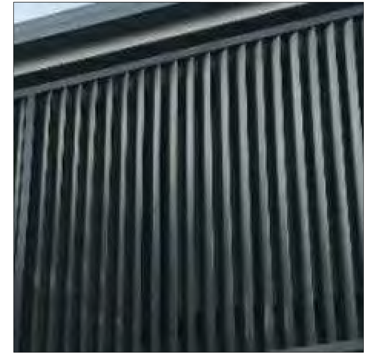
LV - ALUMINIUM LOUVRES IN CHARCOAL POWDERCOATED FINISH
