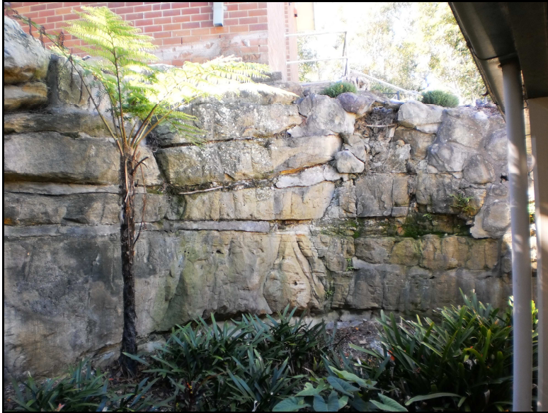
Photograph 1 – Sandstone Cut Supporting Terraced Platform
