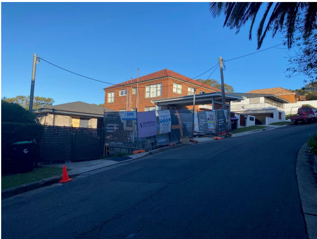
Photograph of the neighbouring property to the south – 8 West Street, Balgowlah
