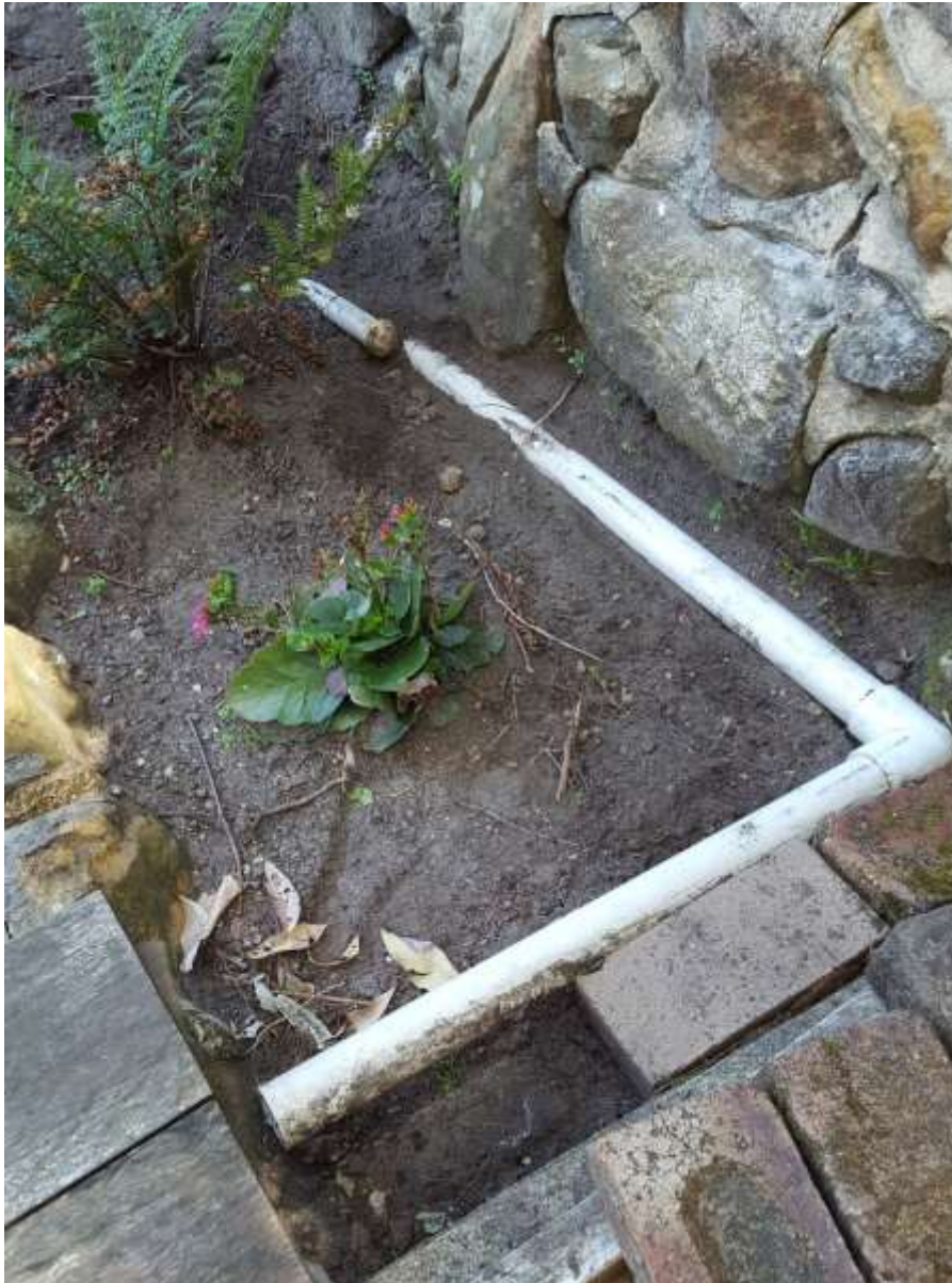
Photo 7 – Additional Pool Plumbing along Boundary Line for Provision of Solar Heating
