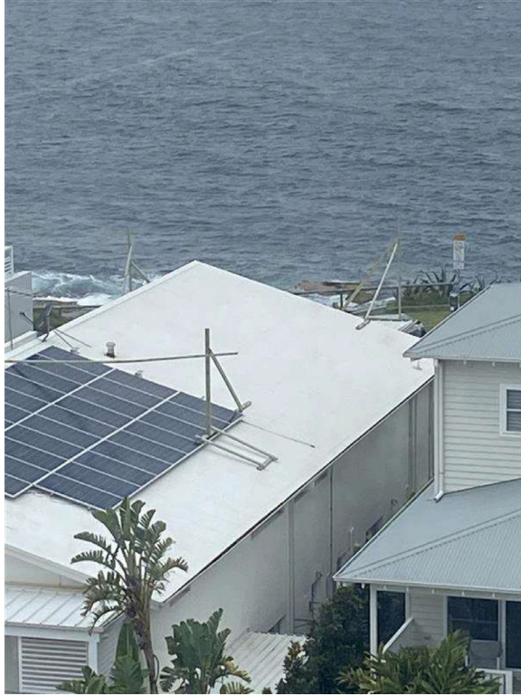
Viewpoint 2: Existing site photo - No.11/186, Pacific Parade.
