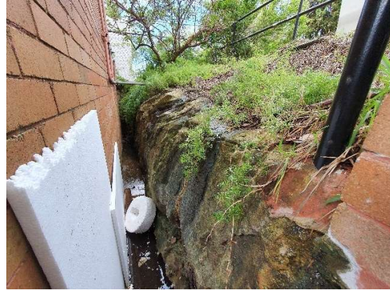
Photograph-12: Low bedrock cutting cliff face. View looking east.
