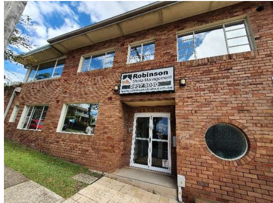
Photograph-14: Building outer wall, facing onto Dowling Street. View looking west.
