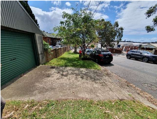
Photograph-8: Dowling Street road reserve, concrete driveway. View looking north.
