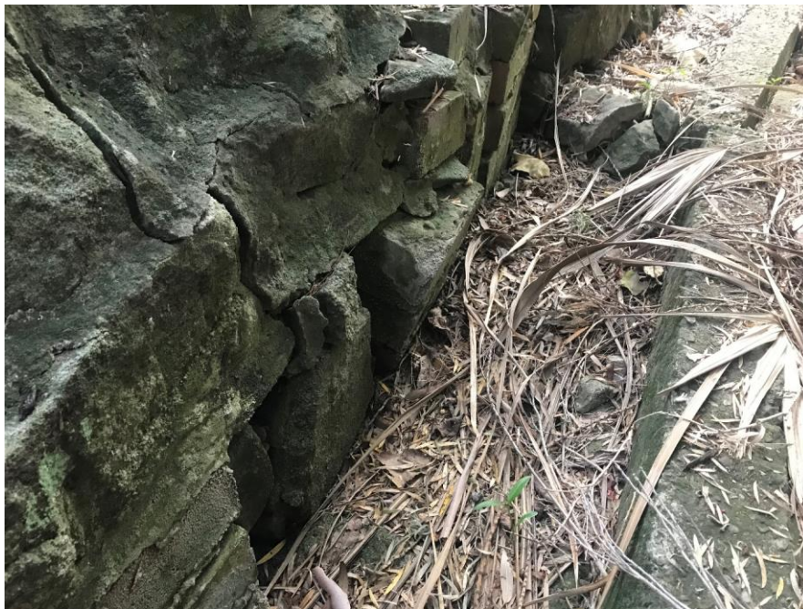
Example of cracking in the existing retaining wall
