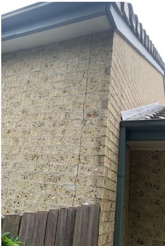
Photograph 3: Vertical crack within rear external wall
